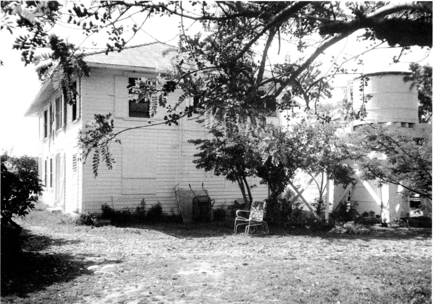
Rear view of the Old Post Office Art Studio; note water tower.
