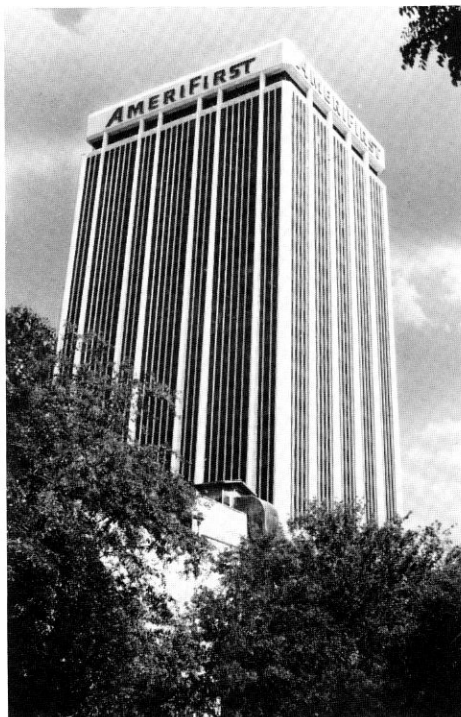
One Southeast Third Avenue, Miami, FL 33131
