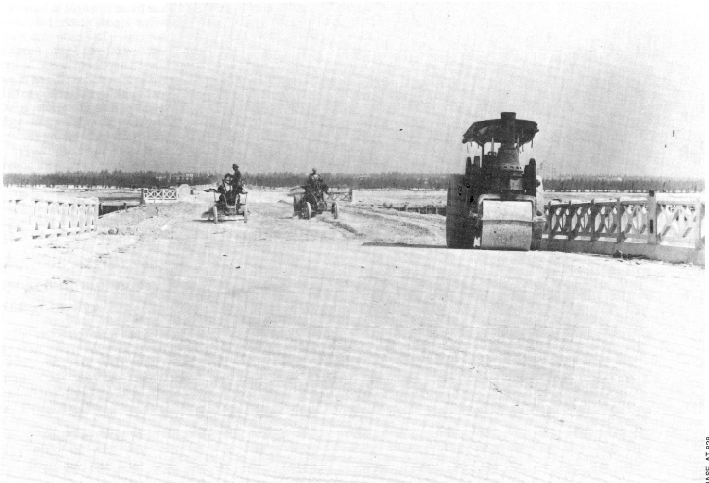
Workers toil in the sun to complete the new macadam-paved Venetian Causeway.
