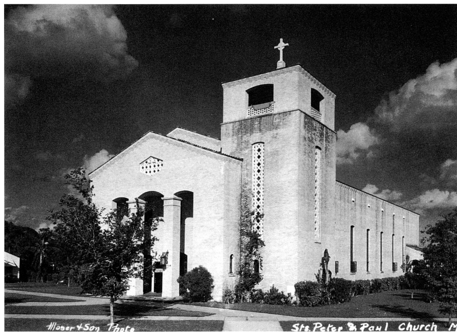
Top—The Warner House, a southern mansion on 111 SW 56 Ave., is one of Little Havana's hidden treasures. HASE, Miami News Collection 1989-011-17920. Above—Sts. Peter and Paul Eastern Orthodox Church on Southwest Tenth Street. Built in the late 1920s, it was at one time the home of John B. Riley, Miami's first mayor. HASE, Miami News Collection 1989-011-3565.
