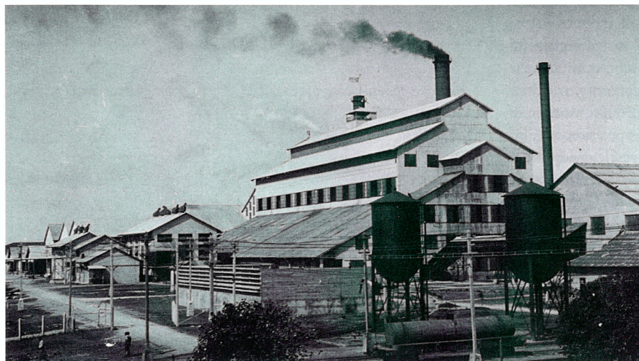
Top—Consolidated Railroads' Budd Rail Diesel Cars leave Havana for Santiago, June 1957 (William D. Middleton). Above—Manatí sugar mill with raw sugar house in foreground, 1920. (Braga Brothers Collection, University of Florida).
