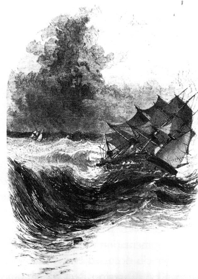
Above—Ship in distress. HASF 82-88-7.
