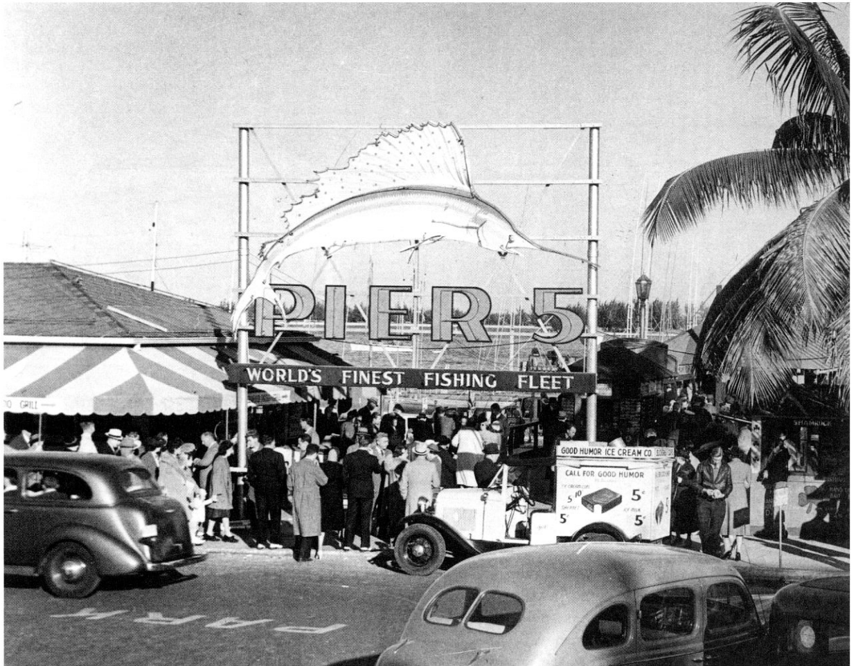
When Bayfront Park was under construction in the early 1920s, Pier Five was rising on its northern edge. HMSF 1982-49-25.
