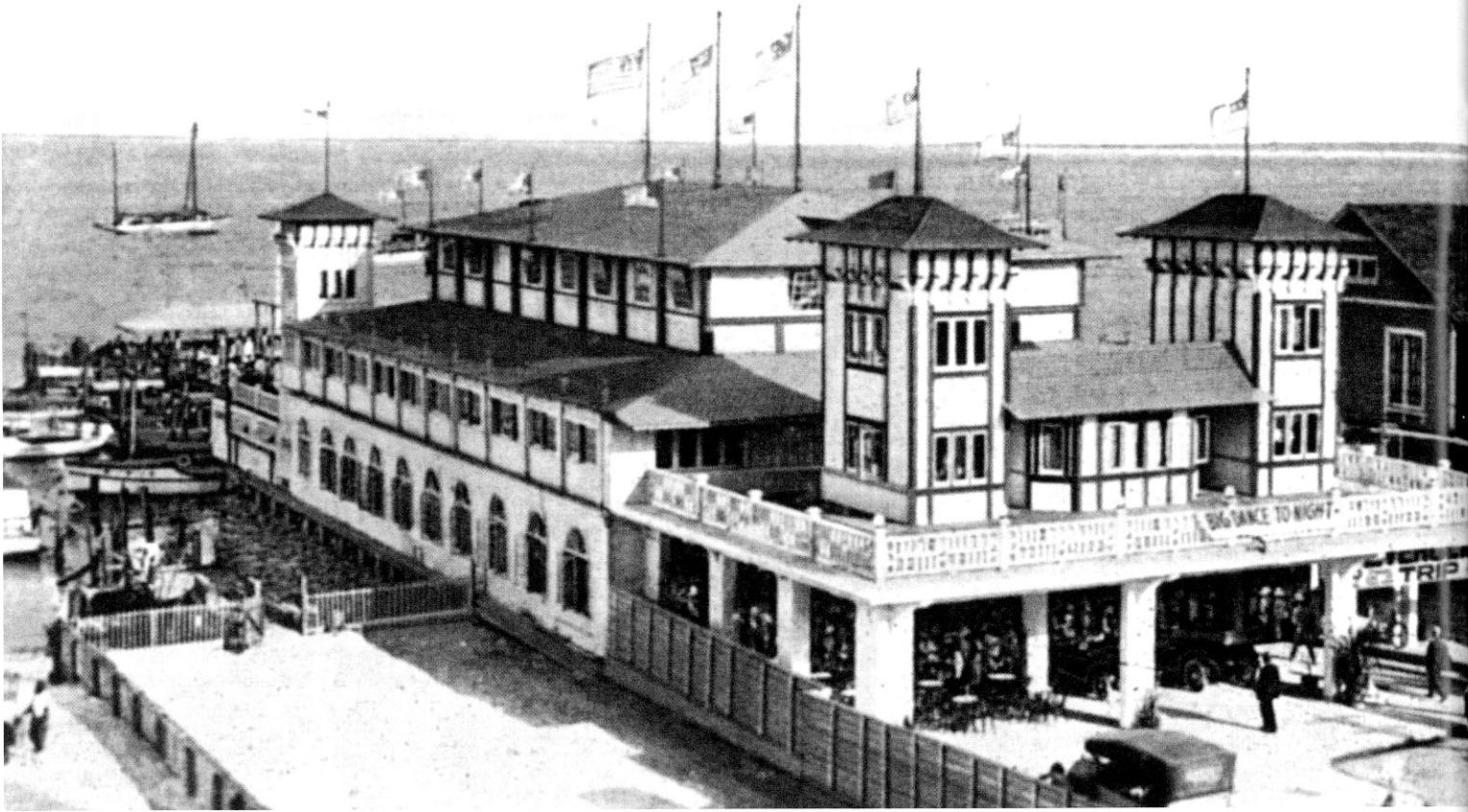
Elser's Recreation Pier, designed by August Geiger, opened at the foot of today's Flagler Street and Biscayne Boulevard in January 1917. HMSF 52-2-74.
