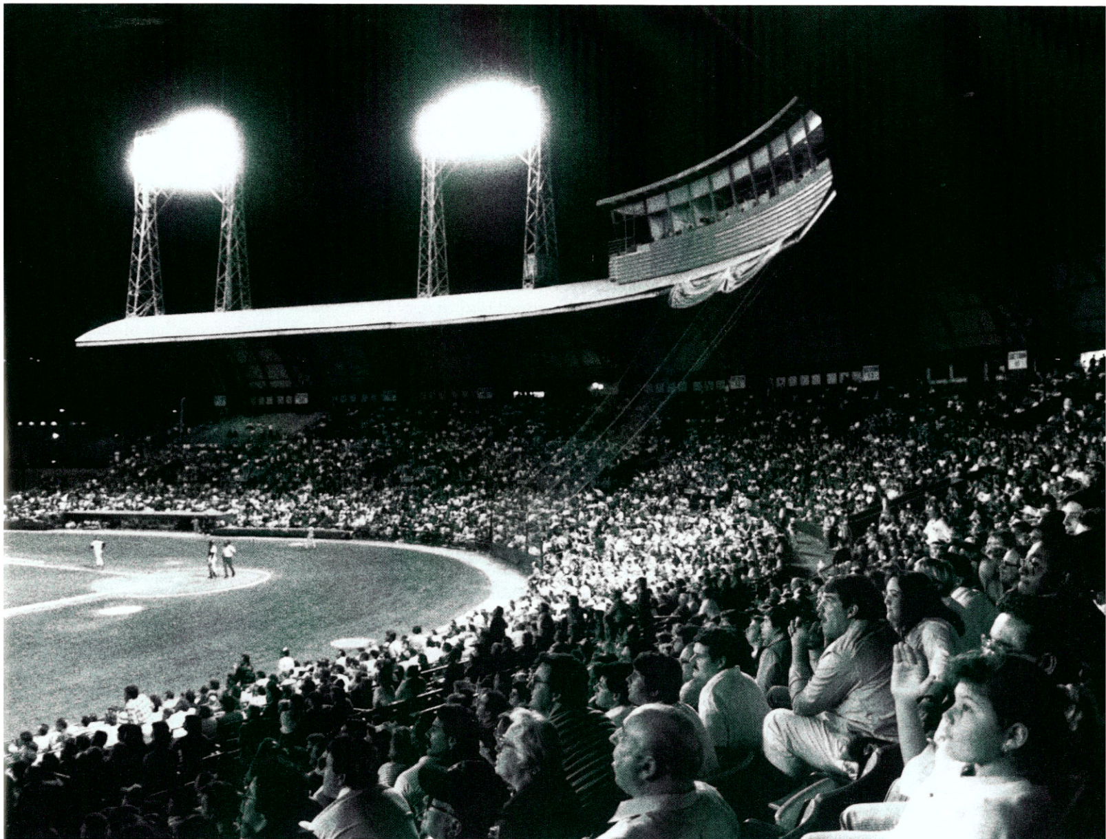
Built in 1949 by Jose Aleman Sr., a onetime, high-level Cuban governmental official, Miami Stadium featured a cantilevered roof and no visual obstructions. For these reasons, the facility, which seated 9,400 fans, was considered state of the art among minor league baseball stadiums. HMF, Miami News Collection 1989-011-15984.
